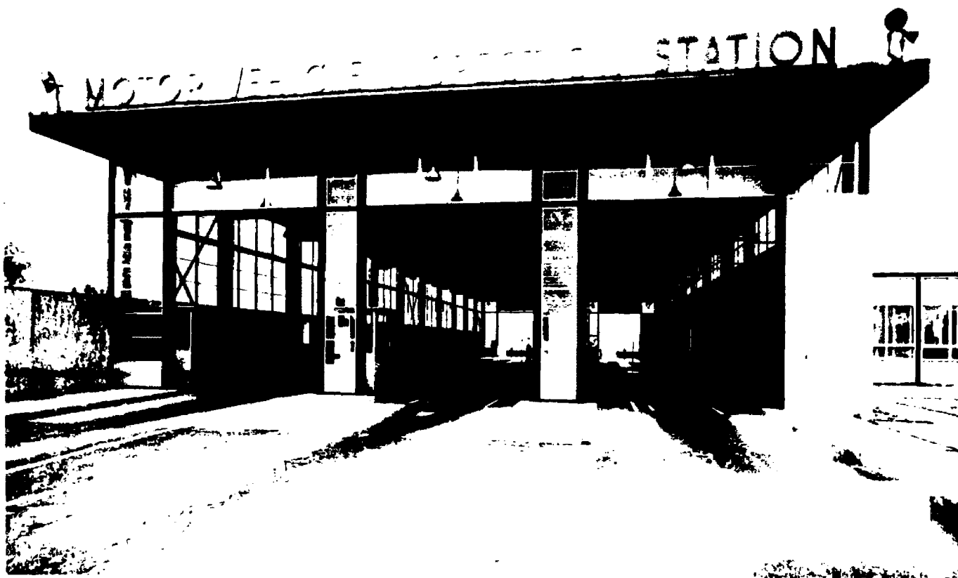
Fig. 8.--State-owned and operated inspection facility in the state of New Jersey.
