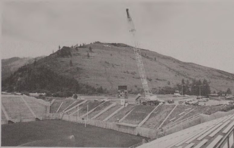
The Washington-Grizzly Stadium expansion project will add 7,000 seats
