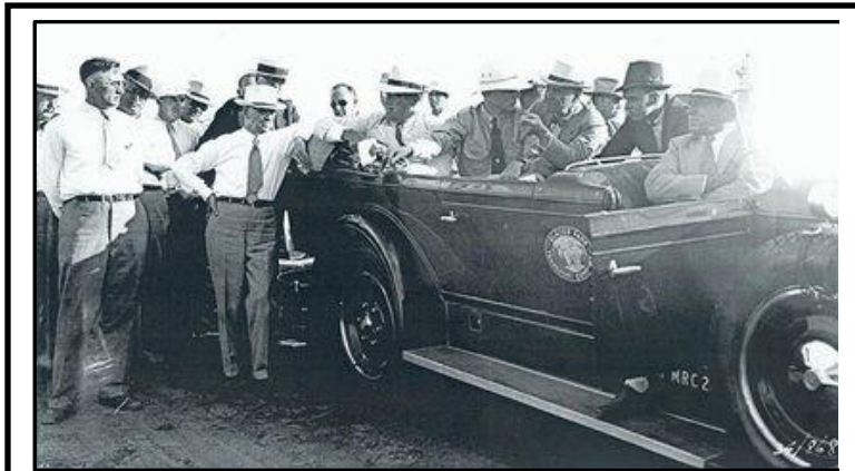
Figure 2. President Roosevelt at Fort Peck Dam Project in 1934 (Gilluly, 2013).
