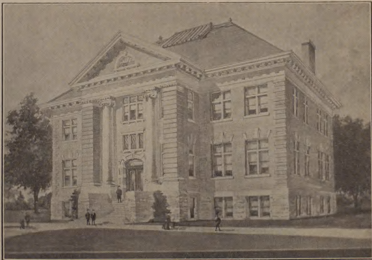
THE LIBRARY BUILDING — IN WHICH THE LAW SCHOOL IS LOCATED
