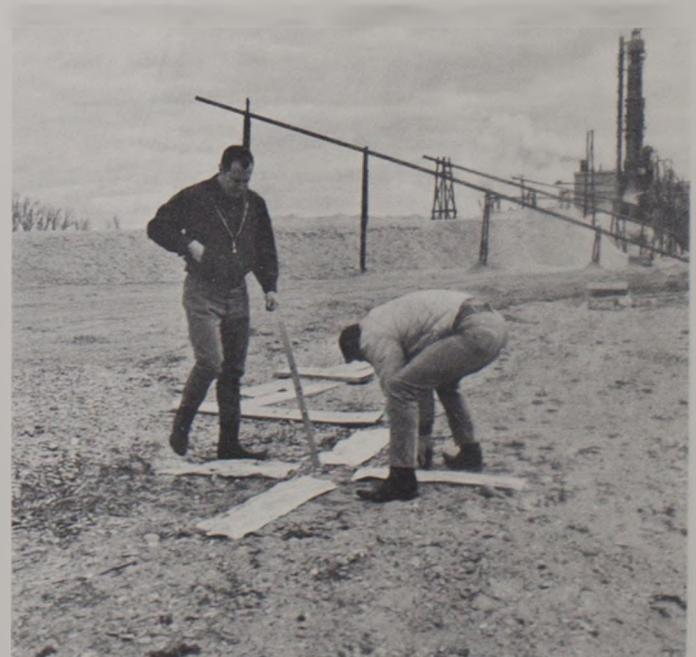
FIGURE 2. Aerial target used for control in the stereo model.
