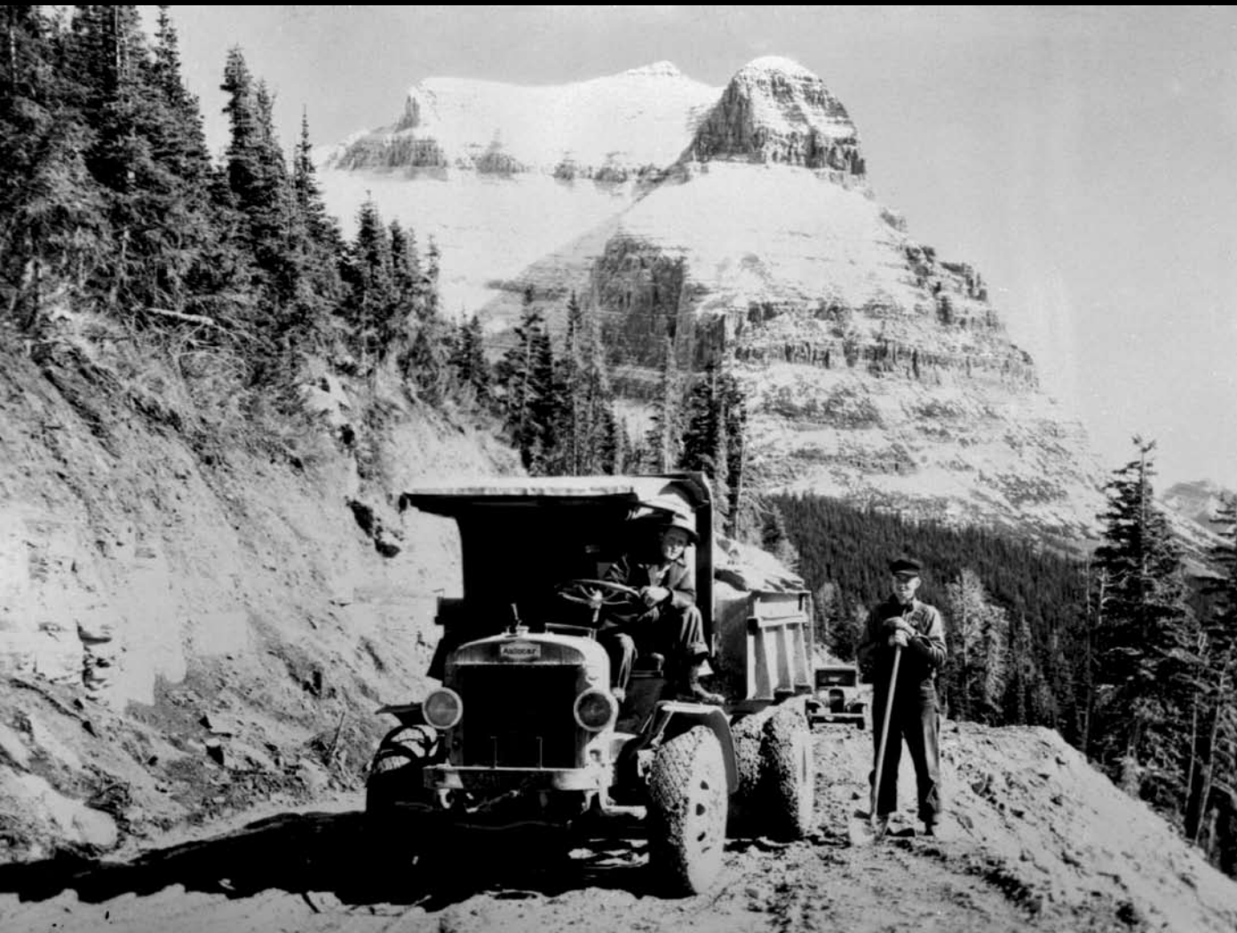
FIRST PAGE: The view of the new Going-to-the-Sun Road in 1934 towards Logan Pass from the west side, just above the loop. (Unknown photographer)
