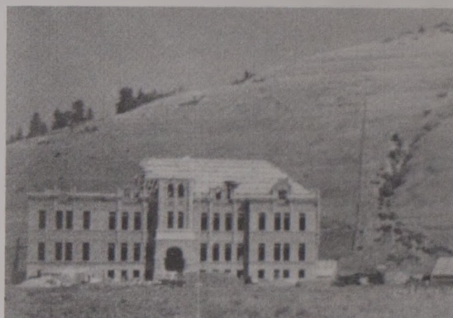
University Hall under construction in 1898 was one of two buildings on campus that year.
