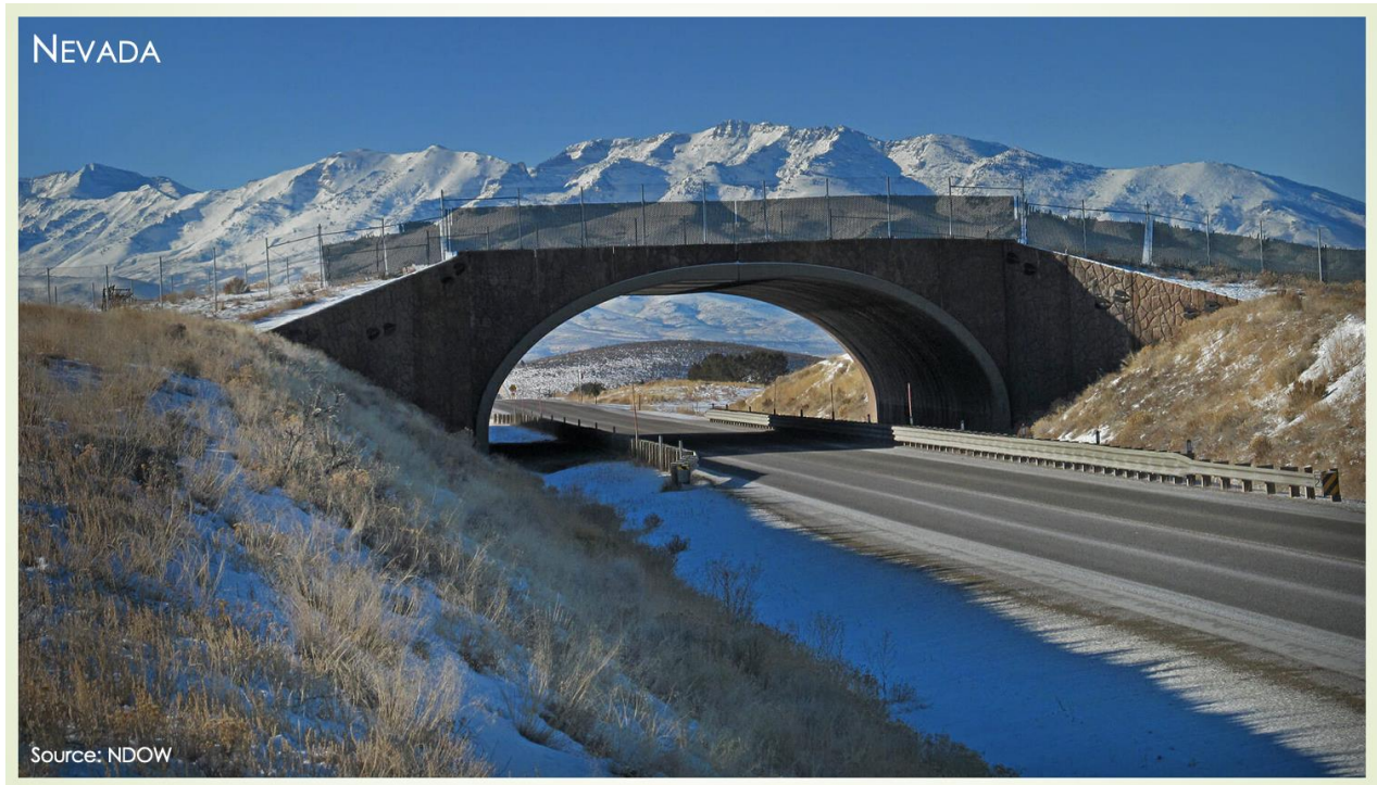
Image 4. A wildlife overpass constructed along Highway 93 in Elko County, Nevada. Source: NDOW.
