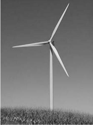
Figure 1. Horizontal Axis Wind Turbine (HAWT).
