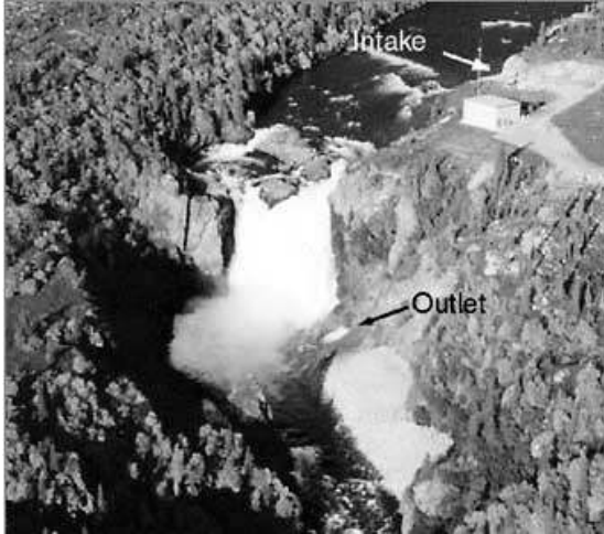
Figure 2. Run of the River Facility (DOE: EERE).
