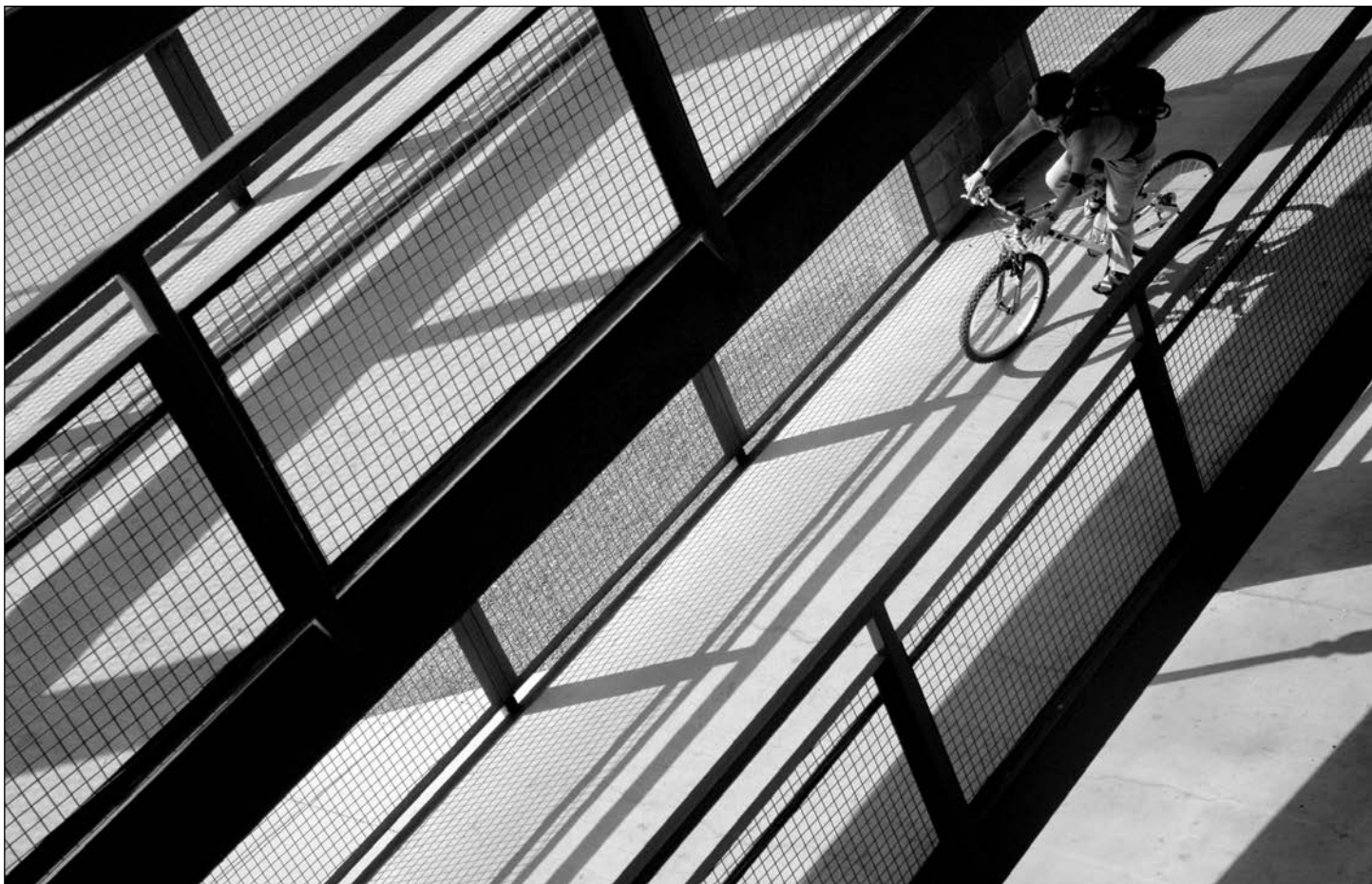
A bicyclist rolls down the south ramp of the pedestrian bridge over the rail road tracks on the edge of downtown Missoula Tuesday afternoon.
