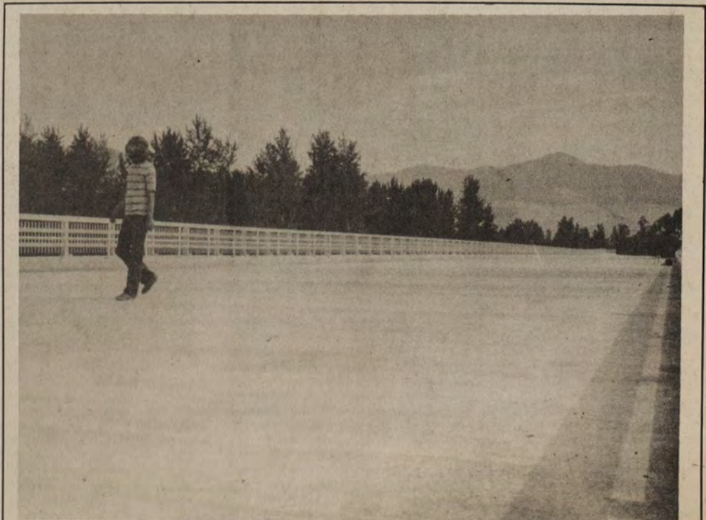
FORMER UM STUDENT BEN FORBES crosses the yet-unsurfaced Reserve Street bridge just west of Missoula. The completed bridge has idly spanned the Clark Fork River since late last year, unused because access roads for the structure have not been built. Construction plans were delayed again Monday when the Missoula County Commission denied permission to construct the access roads in the river's floodplain. (Montana Kaimin photo by Rex Bovee.)
